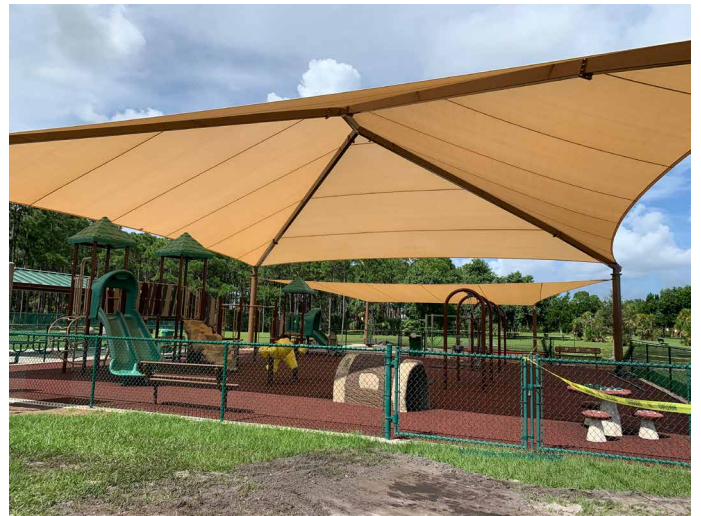
New Shade Structure at Woodland Trails Park
