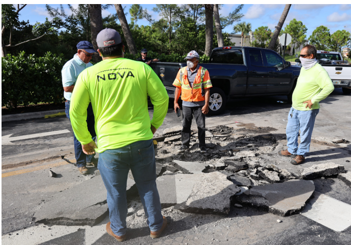
Pioneer Rd Commercial Construction Inspector
