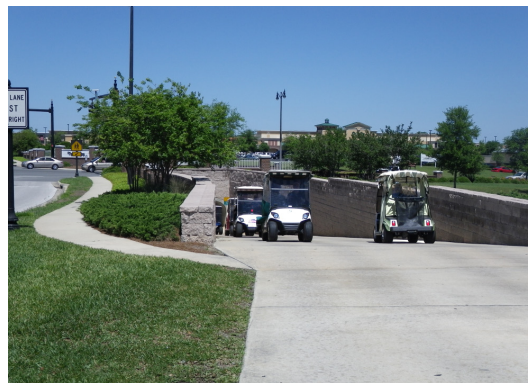
Figure 5 A Golf Cart Trail Underpass in The Villages
