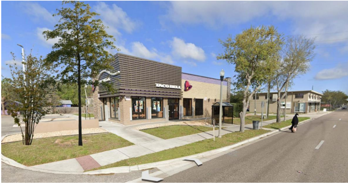
Restaurant with no drive lane in front of building and drive-through at the rear (as currently required by Staff Recc.s)
