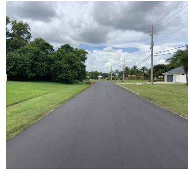
St. Lucie North repaving
