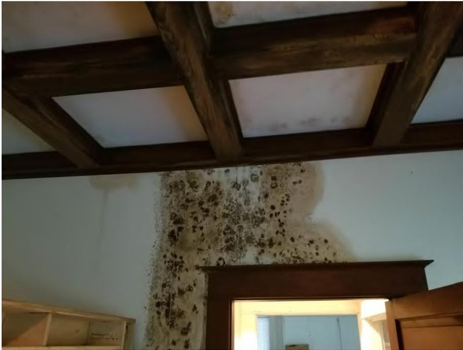
**Photo 5: Water damage and AMG**
