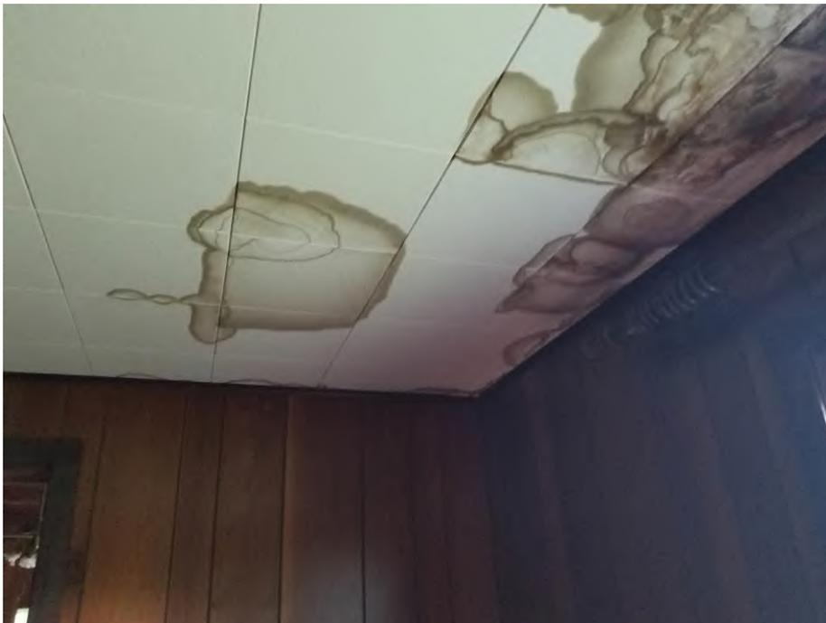
**Photo 12: Water damaged ceiling**
