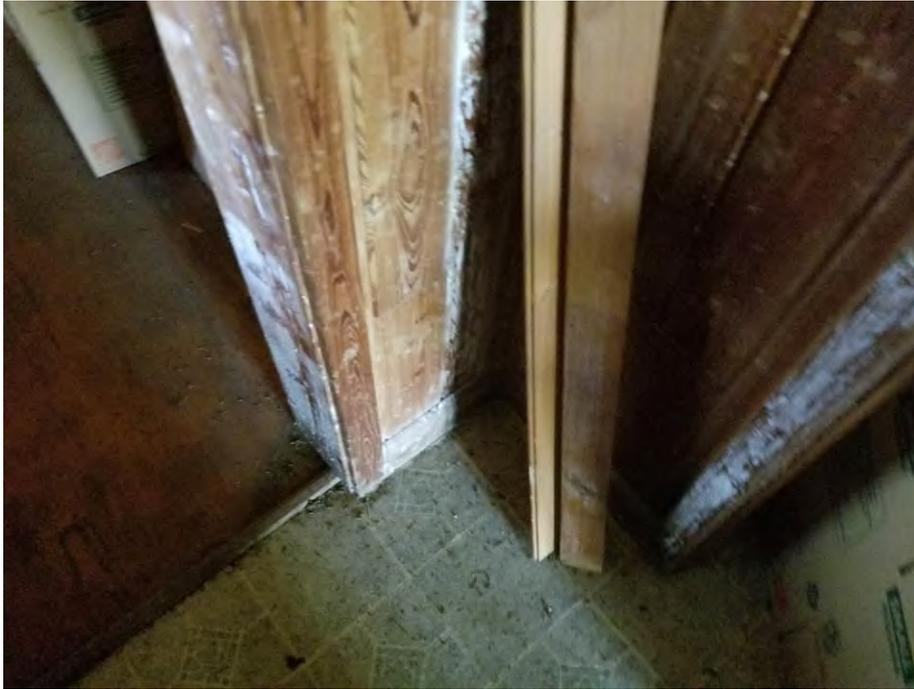
**Photo 11: Water damage and AMG**
