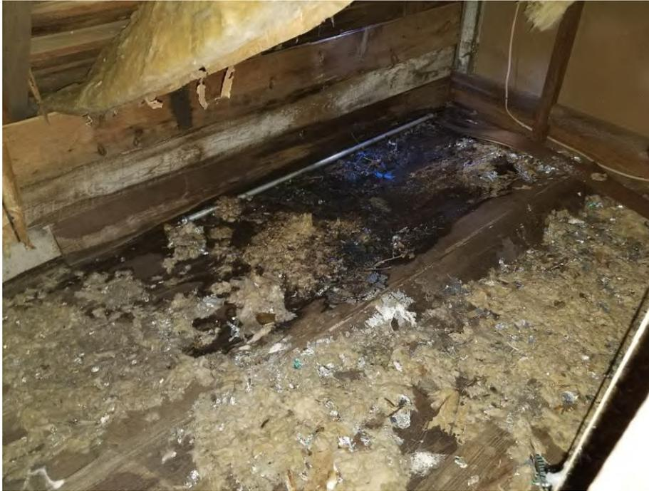
**Photo 7: Water damage and AMG on the second floor**
