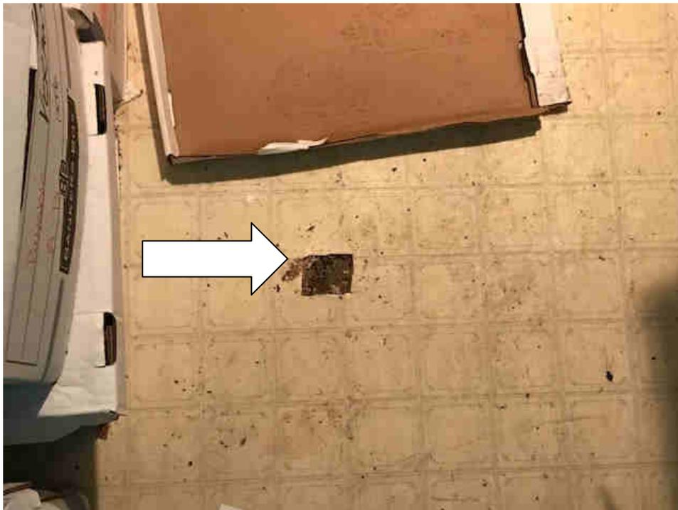
**Photo #1: Typical ACM linoleum flooring in foyer to stairwells – first floor**
