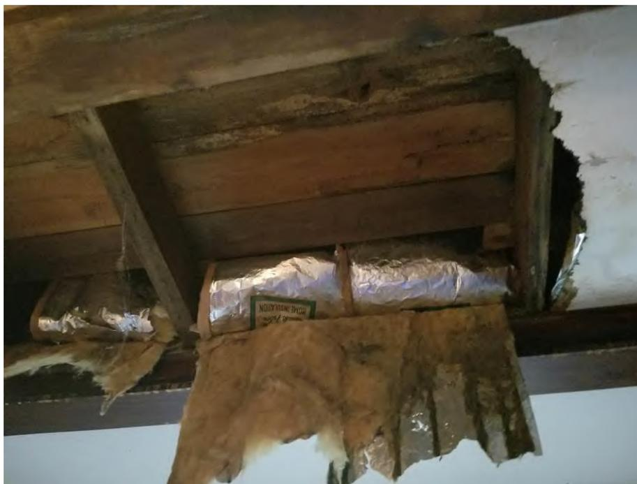
**Photo 4: Typical water damage and AMG on rafters**
