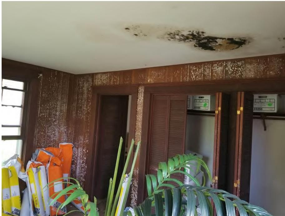
**Photo 3: Water damage and AMG on walls and ceilings**
