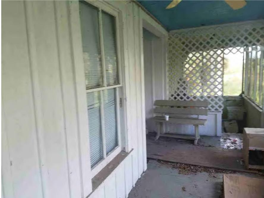
**Photograph #5: Typical view of the typical the exterior walls, ceiling, and windows identified with LBP.**
