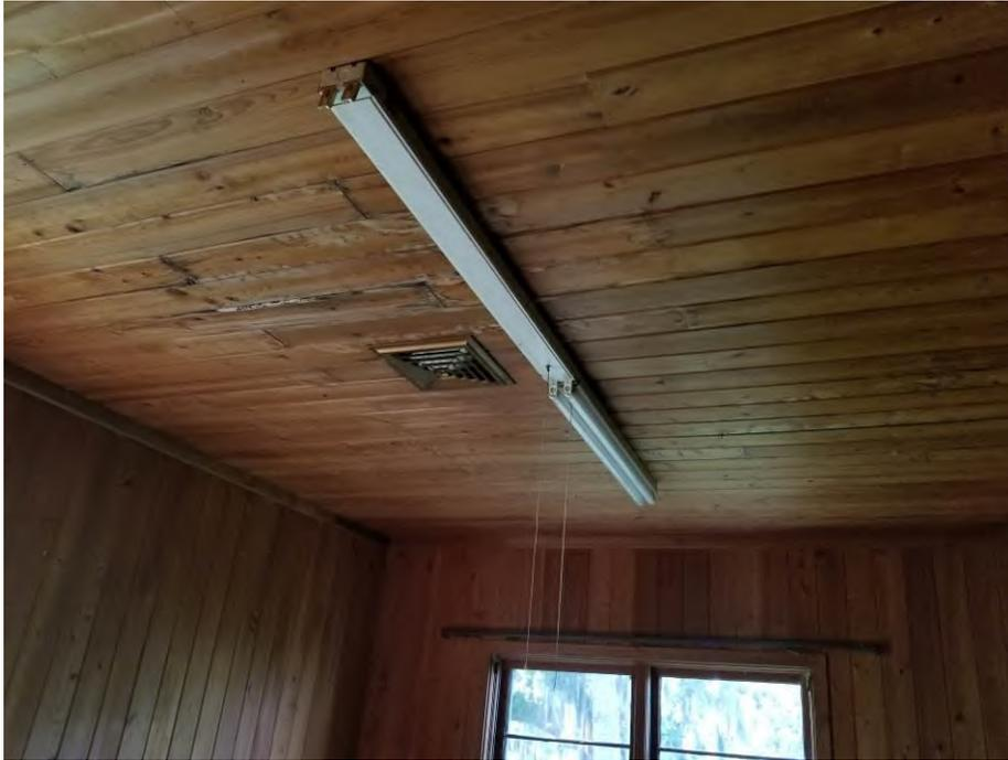
**Photo 13: Water damage and AMG on wood ceiling system**
