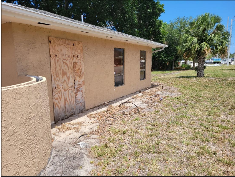
FRONT OF SUBJECT PROPERTY
