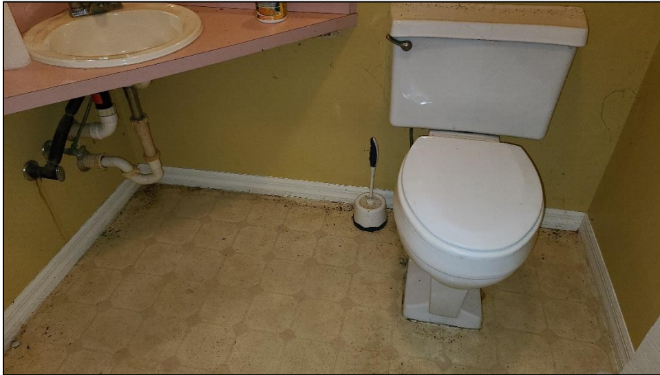
VIEW OF TYPICAL BATHROOM
