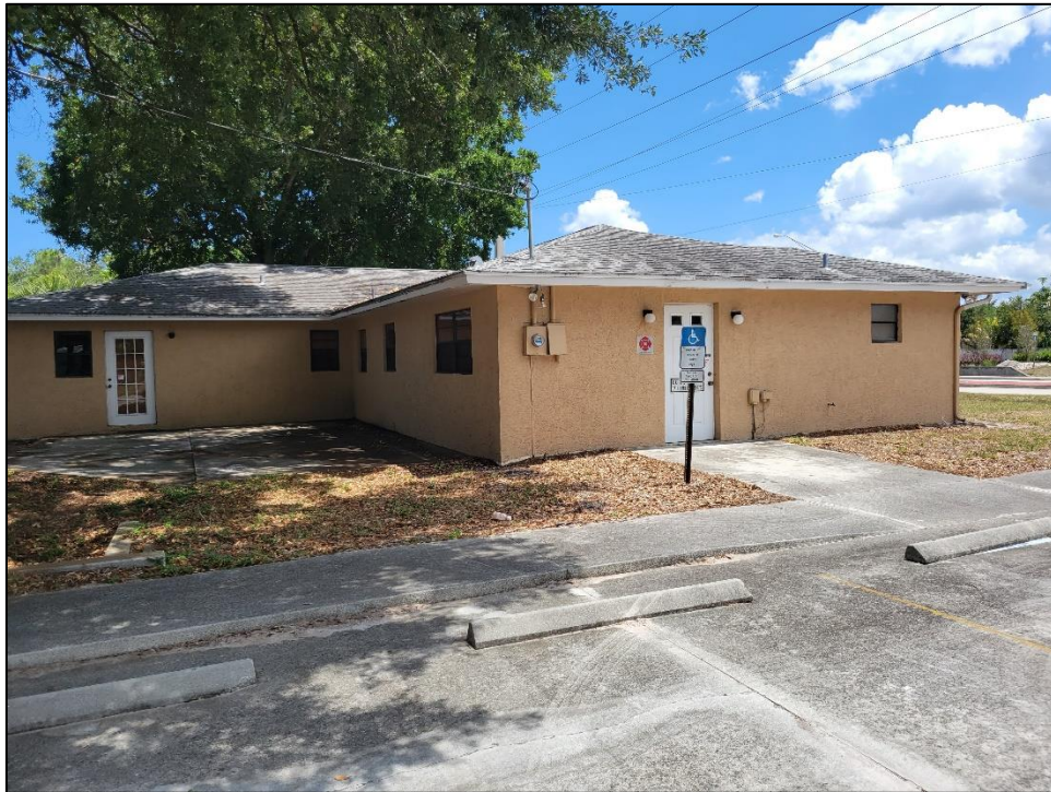
SIDE VIEW OF SUBJECT PROPERTY FROM
