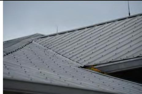
Photo 7.3: Typical roof edge. „V“ crimp system.
