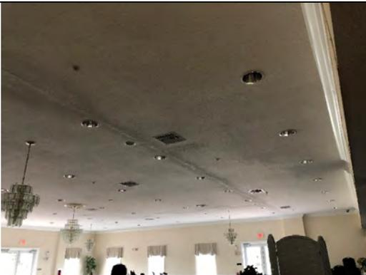
Photo 6.18: Unfinished joint and gaps between exterior plywood ceiling panels
