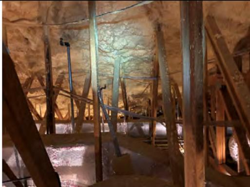
Photo 6.8: Clubhouse wood roof trusses and insulation
