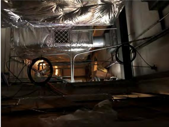
Photo: Gymnasium SE AHU – O/A Intake Ductwork
