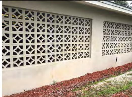
Photo 4.3: Ventilated architectural block and masonry stem wall with open block cells
