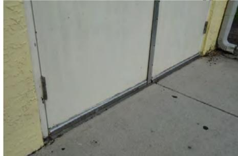
Photo 8.3: Exterior door damage and rust.
