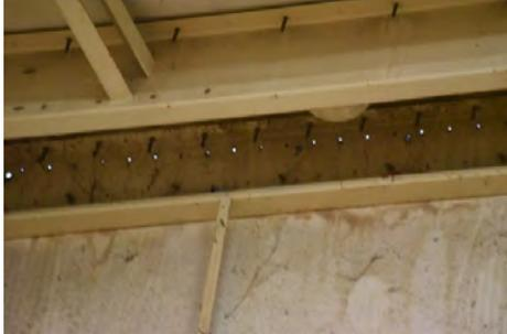
Photo 7.8: Daylight coming in through holes at the roof wall joint.
