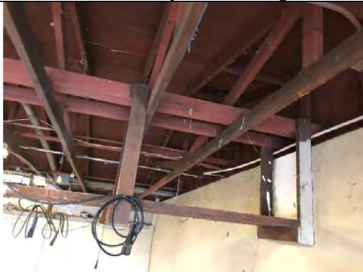
Photo 6.12: Golf Cart building Roof trusses and secondary wood framing
