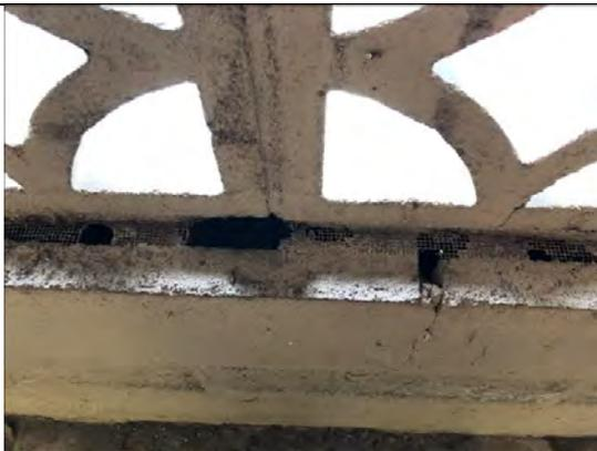
Photo 4.4: Ventilated architectural block and masonry stem wall with open block cells
