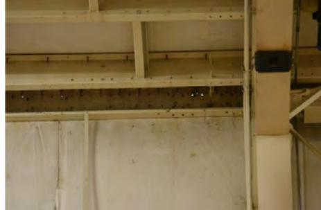
Photo 7.9: Open edges of the roof panels
