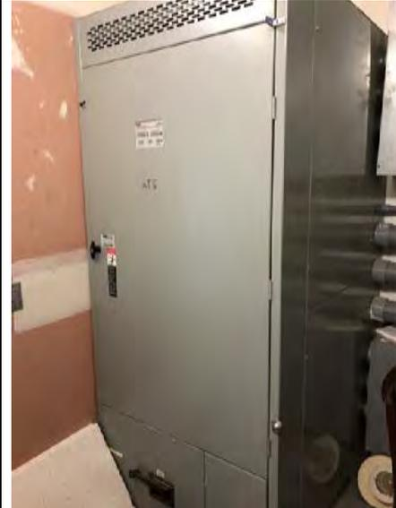
Photo: AC Disconnects – Require Replacing
