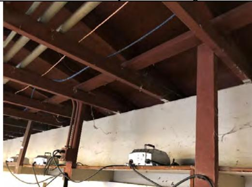
Photo 6.13: Golf Cart building Roof trusses and secondary wood framing and steel I beam with architectural block
