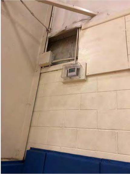
Photo: Gymnasium NW AHU – Thermostat Missing Protective Cover
