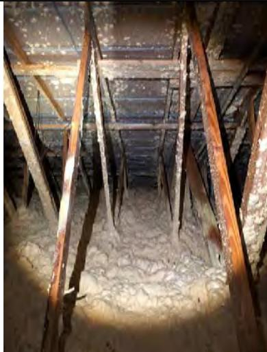
Photo 6.4: Clubhouse wood roof trusses and pipe hanger
