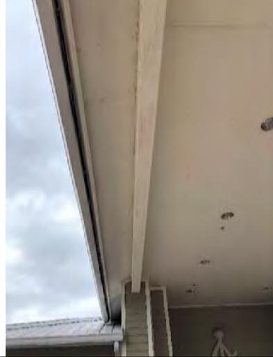
Photo 5.3: Steel beams with some surface rust at the front entrance port cochere
