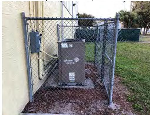
Photo 3.3: Mechanical equipment poured in place concrete pad
