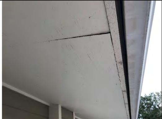
Photo 6.17: Cracked ceiling due to girder truss deflection and movement in the truss to girder truss connection
