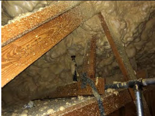
Photo 6.10: Valley piggy back trusses, truss connections
