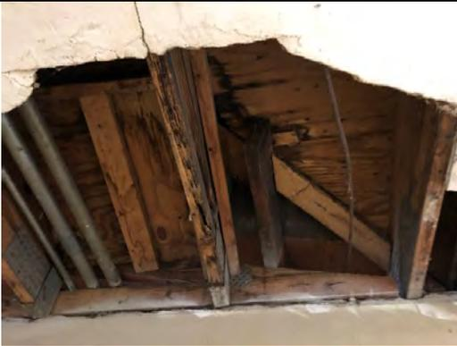
Photo 6.16: Partially detached exterior plywood ceiling panel
