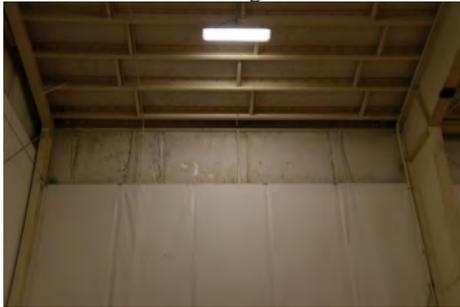
Photo 7.4: Staining of insulation.
