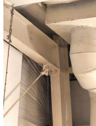
Photo 5.7: Roof purlins and hung mechanical equipment
