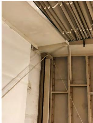
Photo 5.4: Lateral X-Bracing bottom connection
