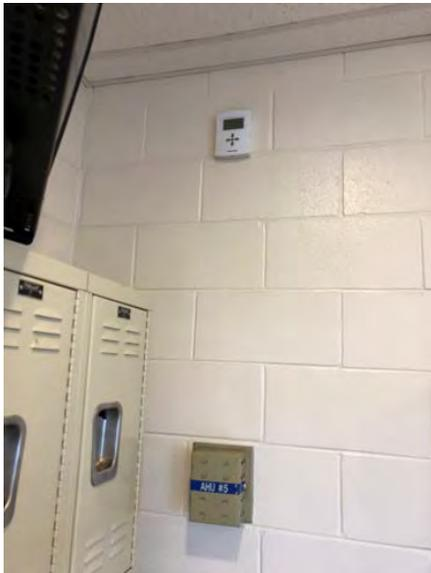
Photo: Gymnasium SE AHU – Thermostat Missing Protective Cover
