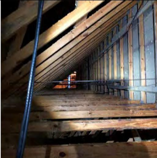
Photo 6.2: Clubhouse wood roof trusses and insulation
