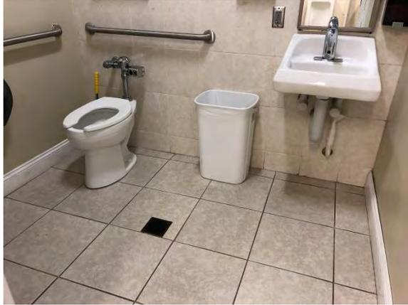
Photo: Flush Valve Water Closet
