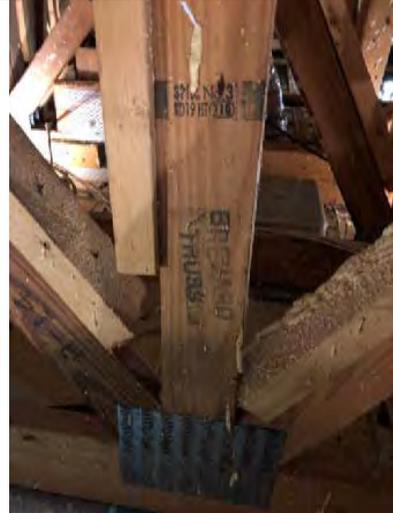
Photo 6.7: Clubhouse wood roof trusses, roof insulation and sprinklers
