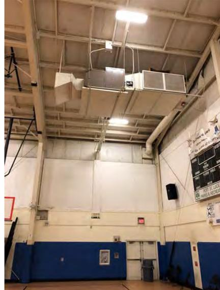
Photo: Gymnasium NW AHU – Sheet Metal Ductwork
