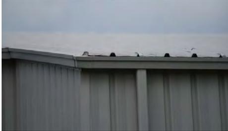
Photo 7.10: Open ends of the roof panels.
