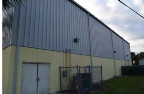
Photo 7.13: exterior metal wall panels.
