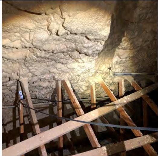
Photo 6.3: Clubhouse wood roof trusses and insulation
