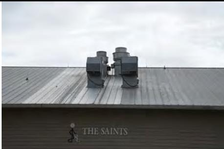
Photo 7.6: Area around the exhaust fans should be cleaned.
