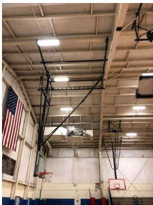
Photo 5.10: Roof purlins and bracing
