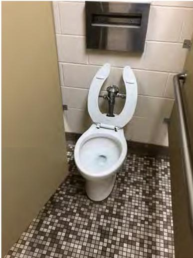
Photo: Flush Valve Water Closet
