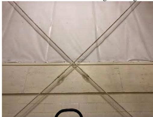
Photo 5.3: Lateral X-Bracing top connection
