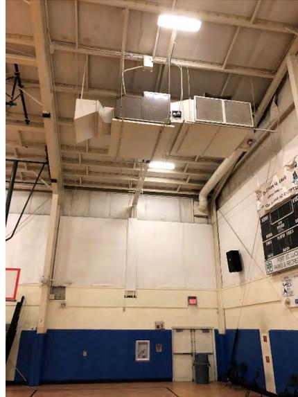
Photo: Gymnasium SW AHU – Thermostat Missing Protective Cover
