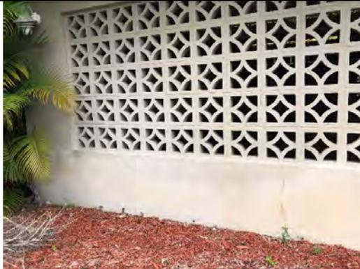
Photo 4.2: Ventilated architectural block and masonry stem wall exhibiting settlement cracks
