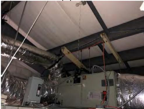
Photo 5.8: Moment Frames, roof purlins and hung equipment platform
