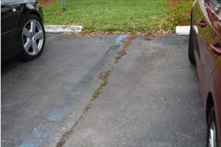
Photo 2.4: Parking lot has some areas of cracking and grass and weeds.
