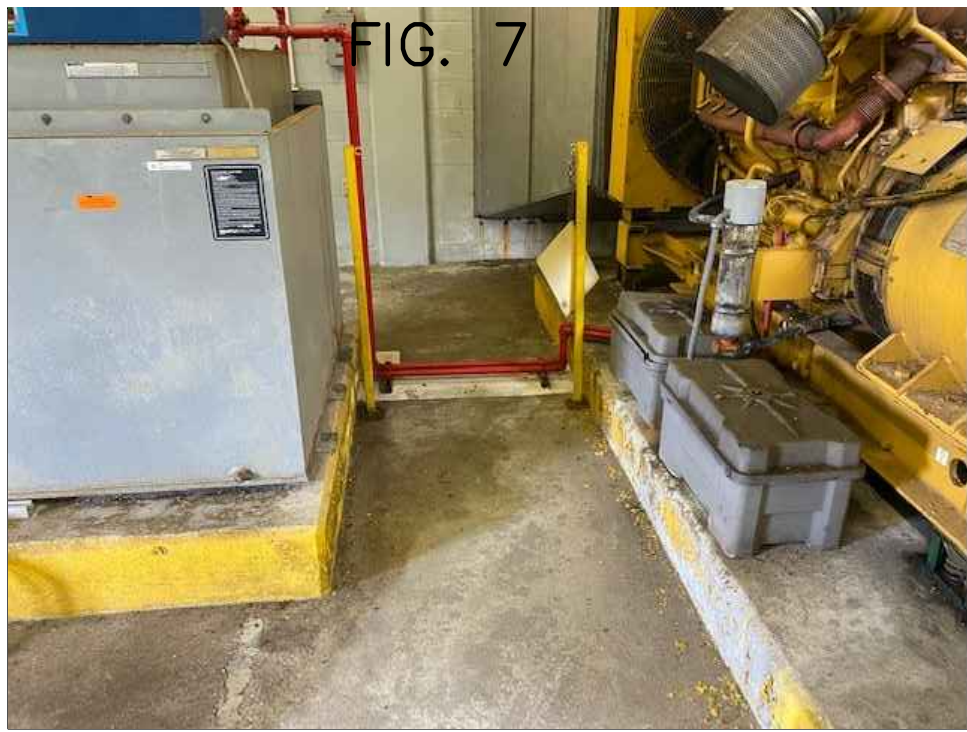
(FIG. 7, 8, 9, 10, and 11) Remove and dispose of existing 300 gallon day tank, existing fuel supply pipes, and fuel return pipes. Remove and dispose of existing electrical conduits & wiring (with exception of fuel sensor blue box and existing generator) in Southport WWTP generator building.
