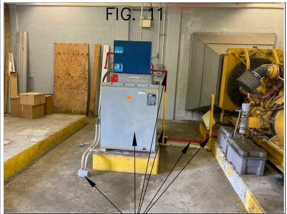
(FIG. 7, 8, 9, 10, and 11) Remove and dispose of existing 300 gallon day tank, existing fuel supply pipes, and fuel return pipes. Remove and dispose of existing electrical conduits & wiring (with exception of fuel sensor blue box and existing generator) in Southport WWTP generator building.
