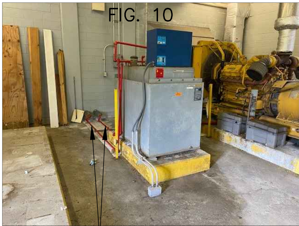
(FIG. 7, 8, 9, 10, and 11) Remove and dispose of existing 300 gallon day tank, existing fuel supply pipes, and fuel return pipes. Remove and dispose of existing electrical conduits & wiring (with exception of fuel sensor blue box and existing generator) in Southport WWTP generator building.
