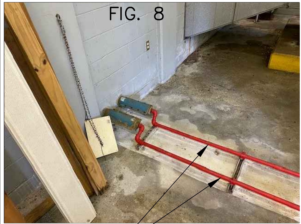
(FIG. 7, 8, 9, 10, and 11) Remove and dispose of existing 300 gallon day tank, existing fuel supply pipes, and fuel return pipes. Remove and dispose of existing electrical conduits & wiring (with exception of fuel sensor blue box and existing generator) in Southport WWTP generator building.
