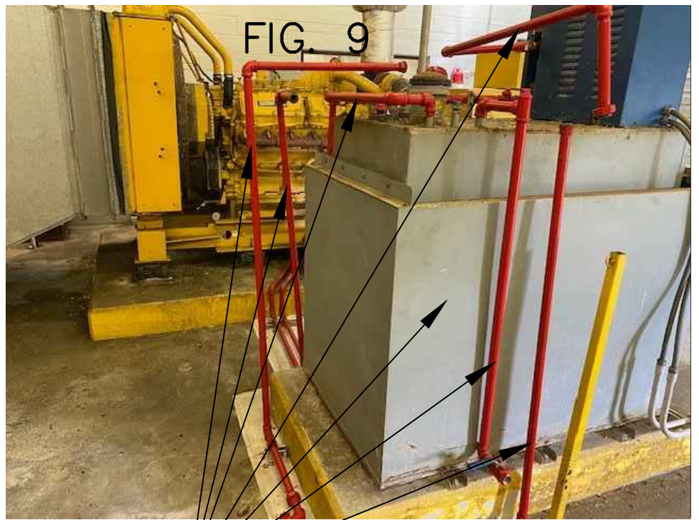
(FIG. 7, 8, 9, 10, and 11) Remove and dispose of existing 300 gallon day tank, existing fuel supply pipes, and fuel return pipes. Remove and dispose of existing electrical conduits & wiring (with exception of fuel sensor blue box and existing generator) in Southport WWTP generator building.
