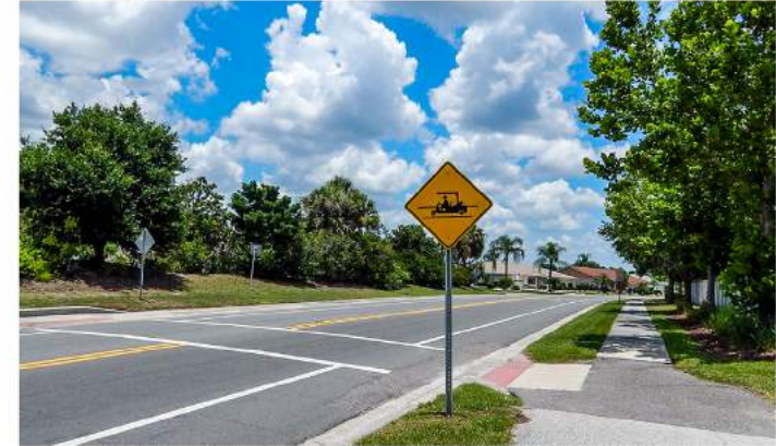
MIDBLOCK CROSSING WITH SIGNAGE - SUN CITY CENTER
