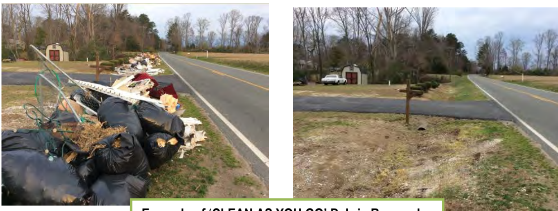
Example of ‘CLEAN AS YOU GO’ Debris Removal
