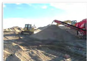
Sand Screening for Renourishment Hurricane Sandy
