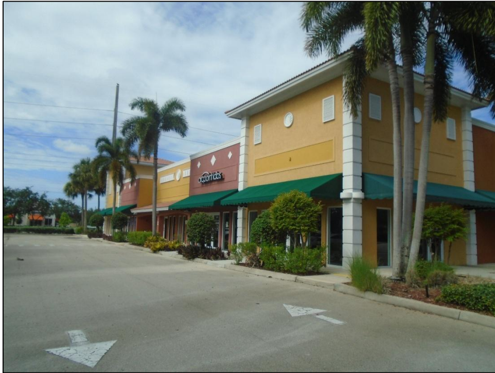
FRONT VIEW OF SUBJECT BUILDING
