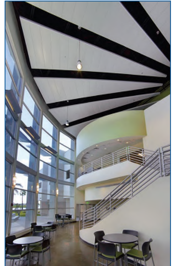
LEED Platinum Certified Palm Beach State College Technical Education Center Belle Glade, Florida
