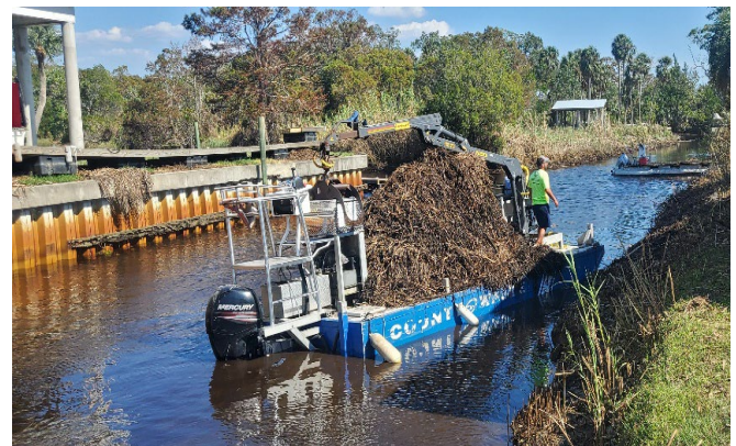
Exhibit 5. Waterway Debris Removal following Hurricane Idalia
