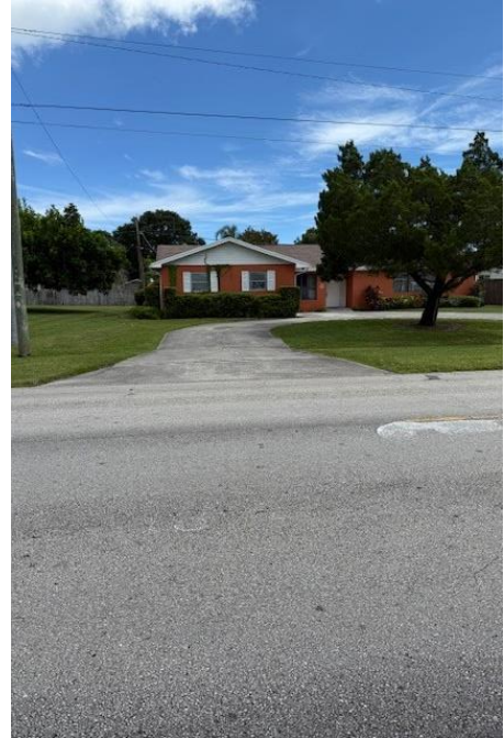
Figure 8 – Driveway Tie-in Issues
