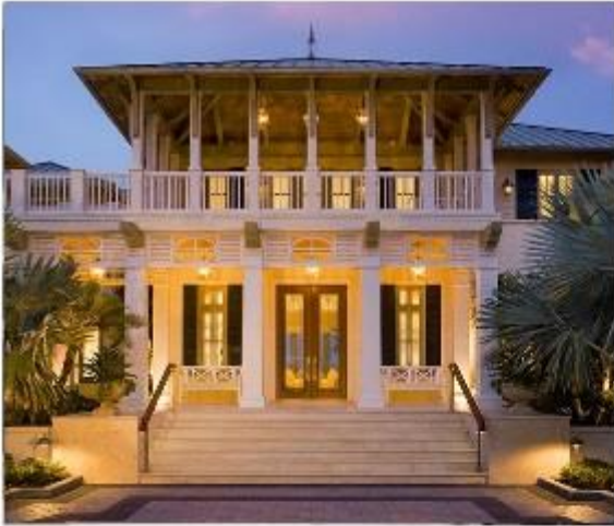
Figure 4-3: Examples of Florida Vernacular Style (continued)
