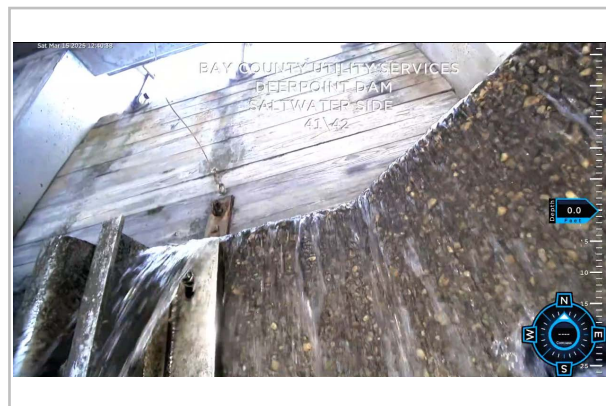
Broken Lifting Cable (44/45)
