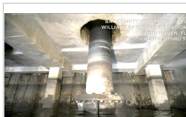
Corrosion & Growth (Pump 2)
