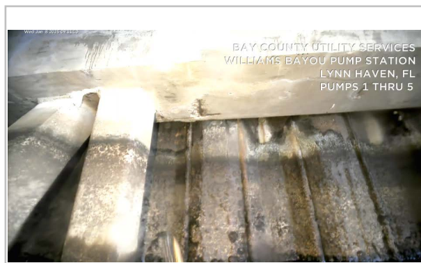
Exposed Reinforcement - Header Near Pump 1
