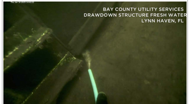
Leak (Flapper Gate 10)
