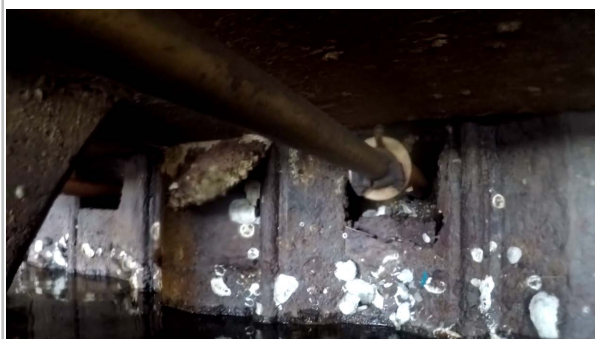
Corrosion & Tieback Void (56/ Abutment)
