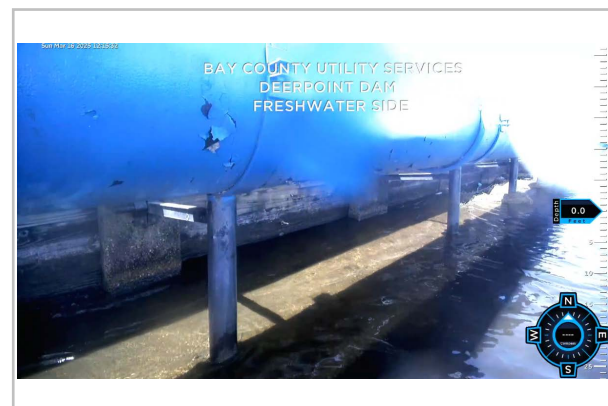
Freshwater Stuck Float and Debris
