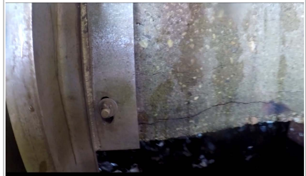
Loose Eye Bolt (56 Abutment)
