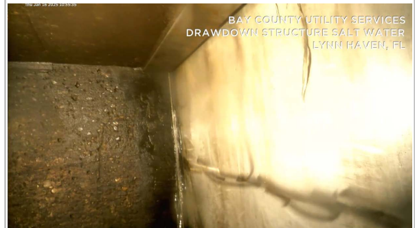
Heavy Exposed Aggregate (Wall)
