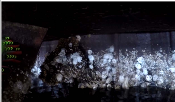
Corrosion & Tieback Void (56/ Abutment)
