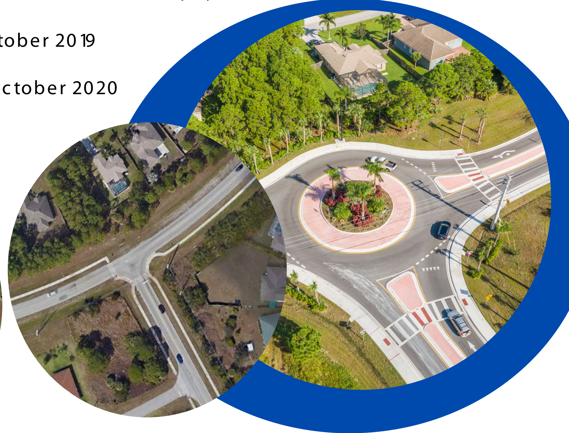
East Torino Pkwy and SW Cashmere Blvd Roundabout Project
