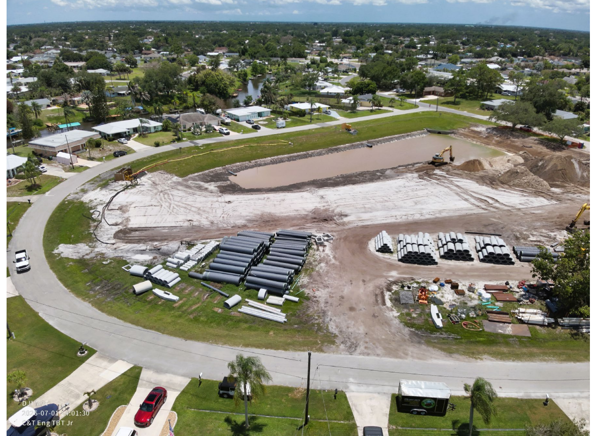
Harbour View Stormwater Pond Activities
