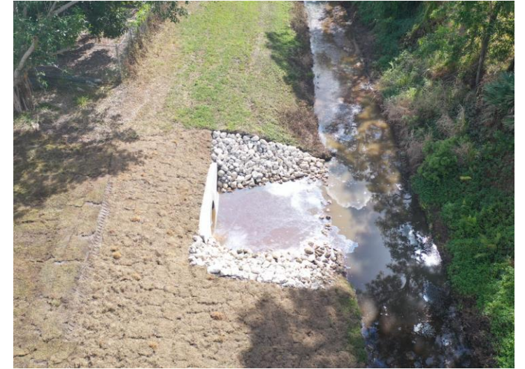
Walters Terrace Pond Outfall
