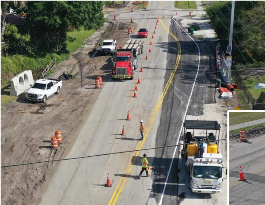
Lane Shift for Drainage Crossing Replacement
