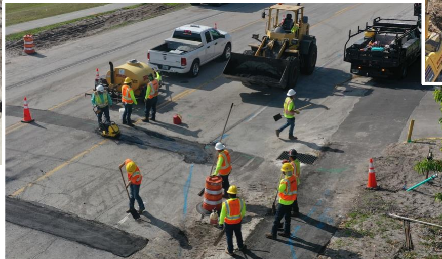
Installing Utility Crossings
