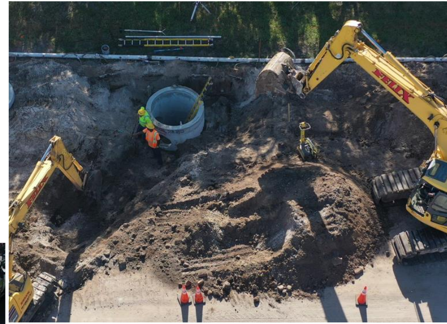
Installing Drainage Structure
