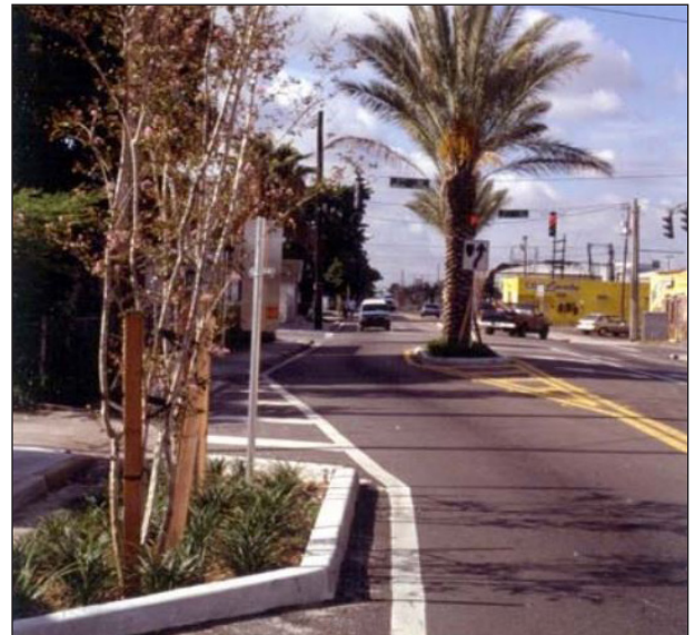
Bulb-out and median create a lateral shift in the travel route. Image courtesy of Ian Lockwood.
