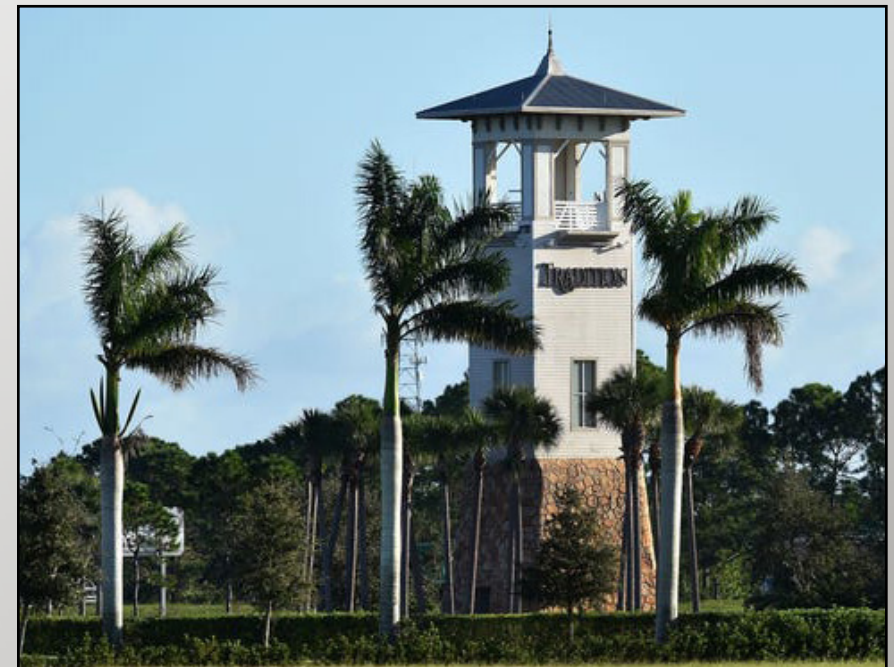
Figure 53 The Tradition DRI has employed a signature tower design to brand the community. Credit: TCPalm
