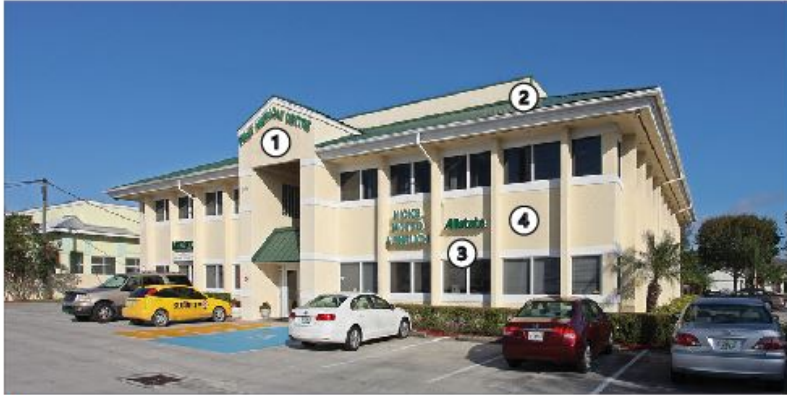
TWO STORY OFFICE BUILDING
