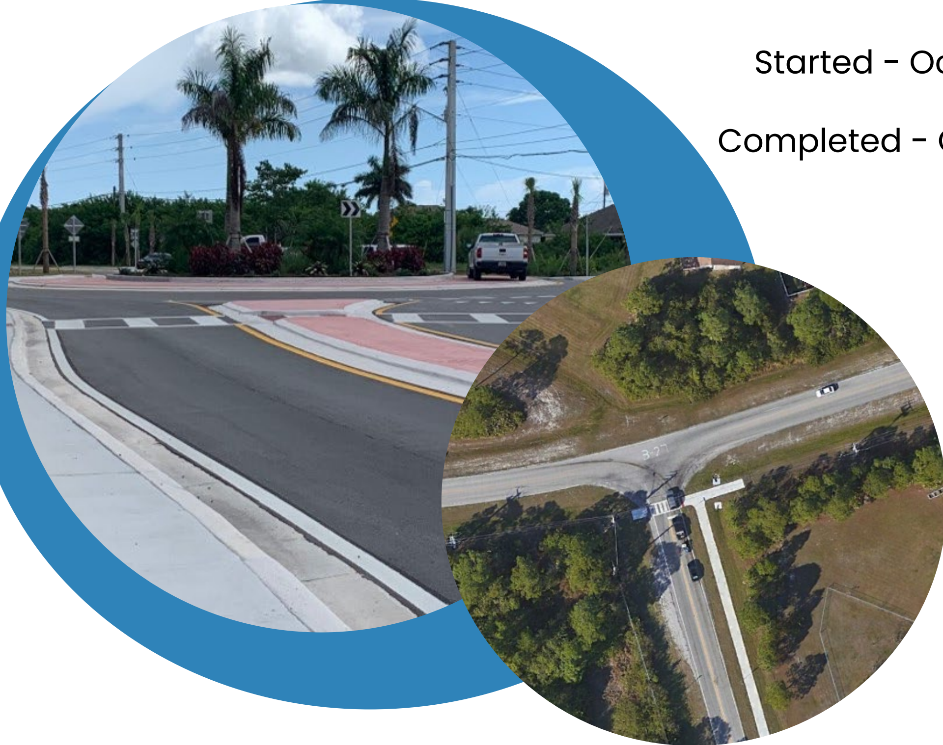
East Torino Pkwy and NW California Blvd Roundabout Project
