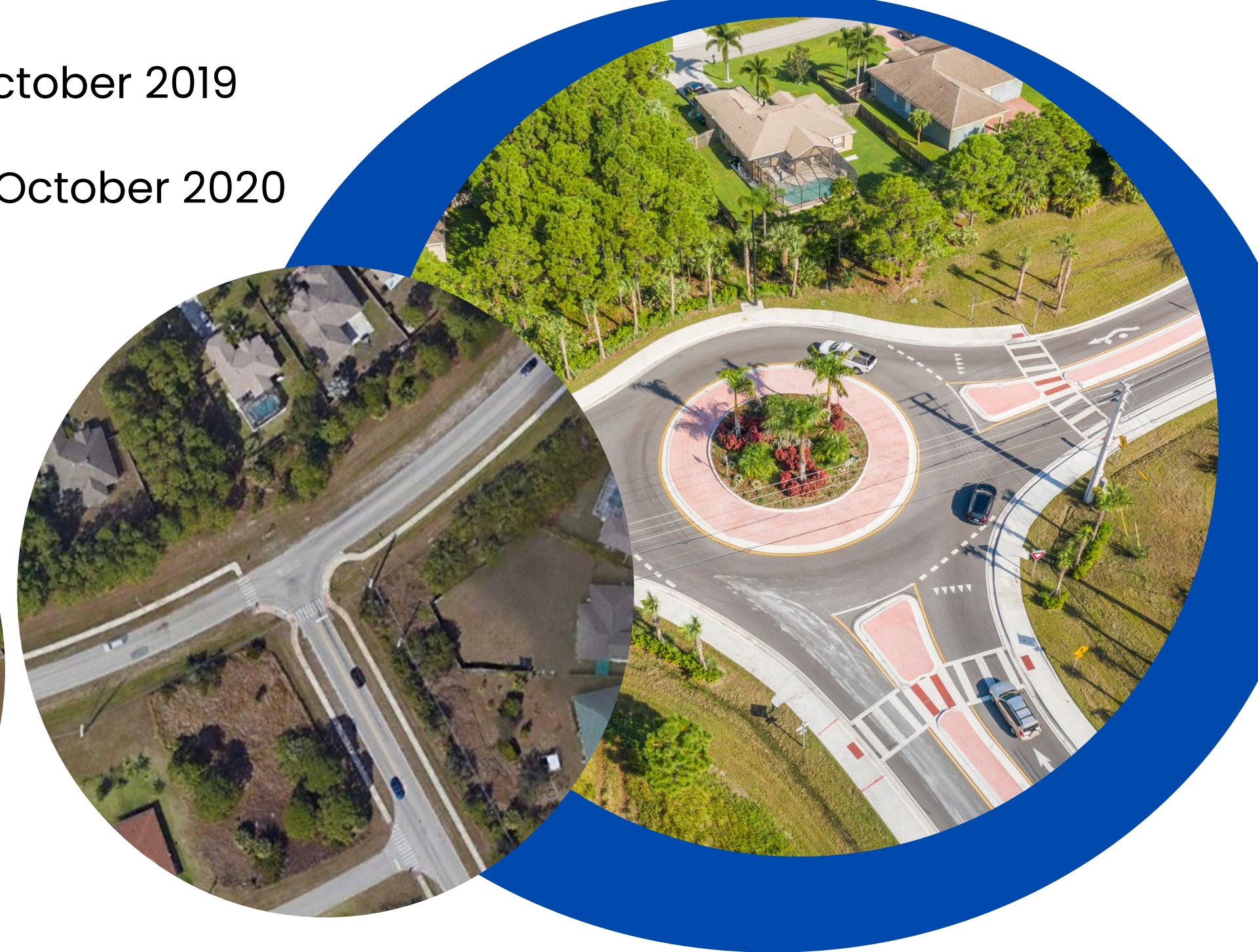
East Torino Pkwy and SW Cashmere Blvd Roundabout Project
