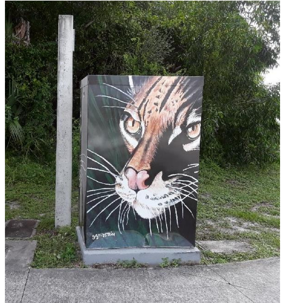
Utility Box Wrap – NE corner of Airoso Boulevard & Floresta Drive
