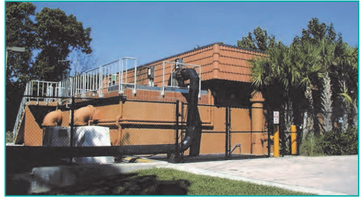
Figure 5. Aesthetics are always considered in designing pump stations, with structures built either underground or in harmony with their neighborhoods. (Collier County Master Pump Station).
