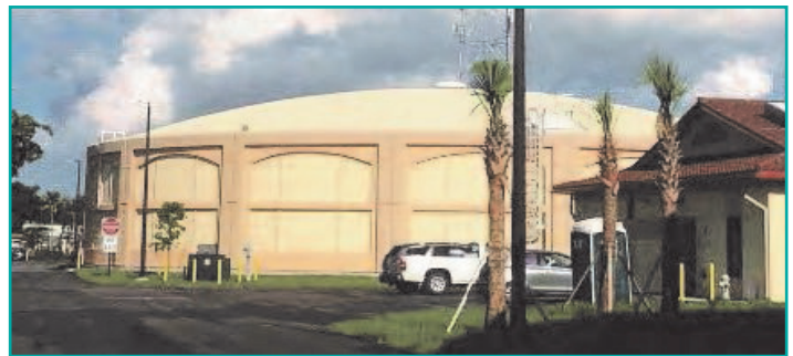
Figure 20. AECOM provided for localized hydraulic modeling and calibration to provide set points for remote system operations' optimization for West Hollywood pumping and storage facility.
