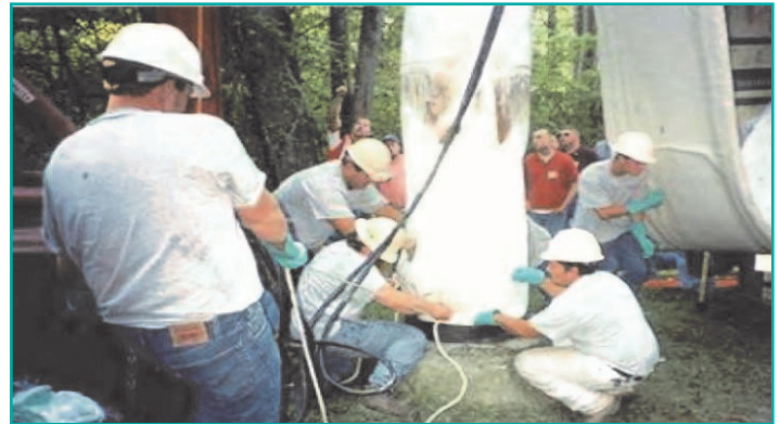
Figure 12. PVC Pipe Lining, Sewer Rehabilitation, North Miami Beach, FL.
