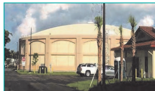
Figure 7. The West Hollywood Pumping Station and Storage facility includes two 2.5-mg aboveground storage tanks.
