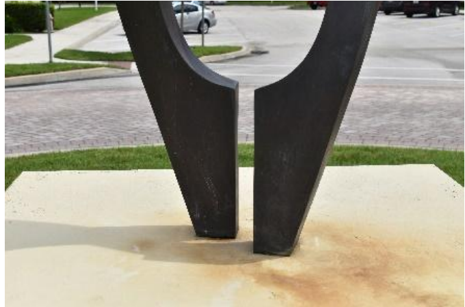
Figure 26. Corrosion on vertical surface of bronze sculpture and possible evidence of blanching wax. Residual staining is visible on the top face of the concrete base (Photo by EverGreene, October 2022).
