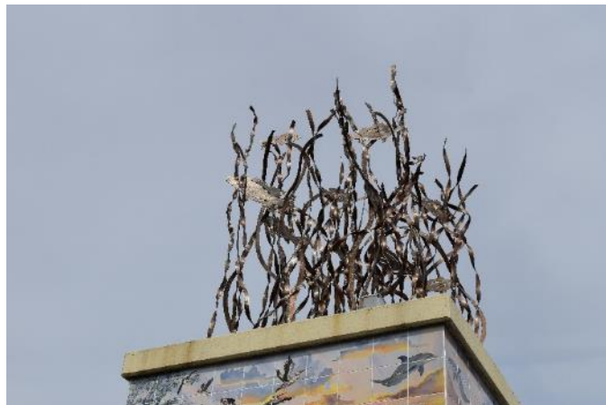
Figure 91. Discoloration of the metal sculpture with corrosion product streaked down the face of the concrete border to the tiles. It is unclear if this residue reached the tiles below (Photo by EverGreene, October 2022).
