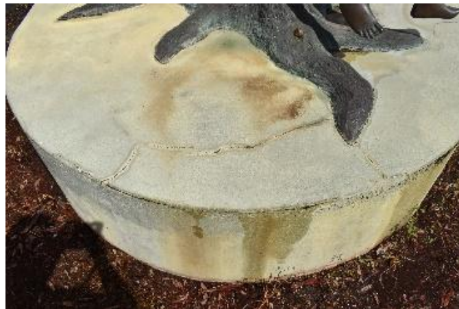
Figure 7. Major cracking from the base of the sculpture across the top face of the concrete base (Photo by EverGreene, October 2022).
