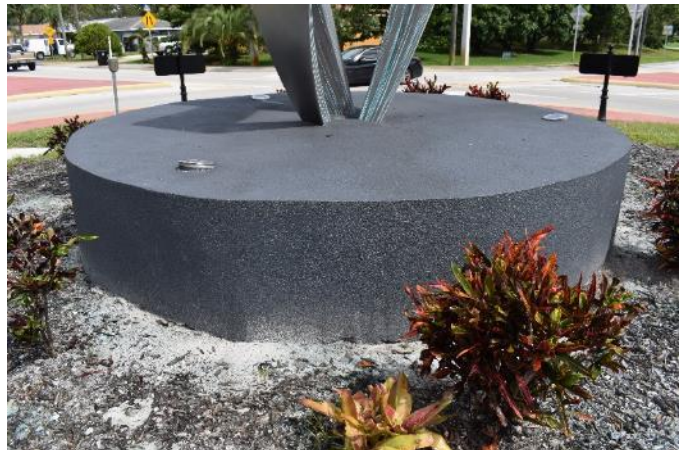
Figure 121. Dirt or sand accumulation at the bottom of the concrete base (Photo by EverGreene, October 2022).
