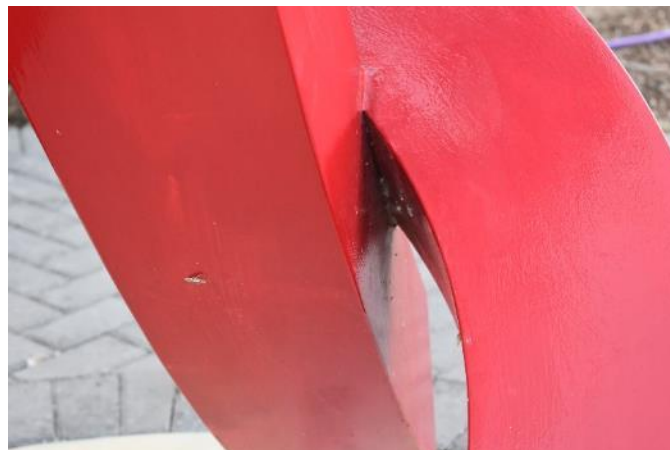
Figure 82. Debris and organic material buildup within a joint between two sculptural elements (Photo by EverGreene, October 2022).
