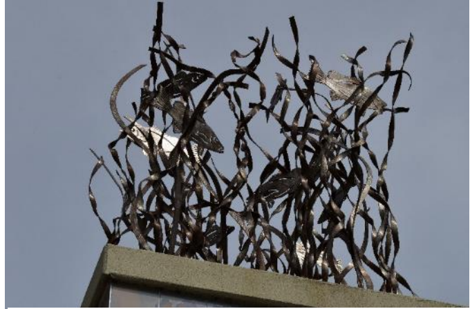
Figure g3. Detail image of the metal sculpture. There is minor residue staining on the ledge above the tiles (Photo by EverGreene, October 2022).
