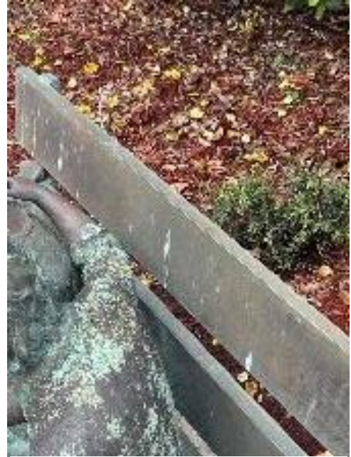
Figure 11. Green corrosion on the figure of the boy. Animal guano and staining is visible on the front of the bench back support (Photo by EverGreene, October 2022).
