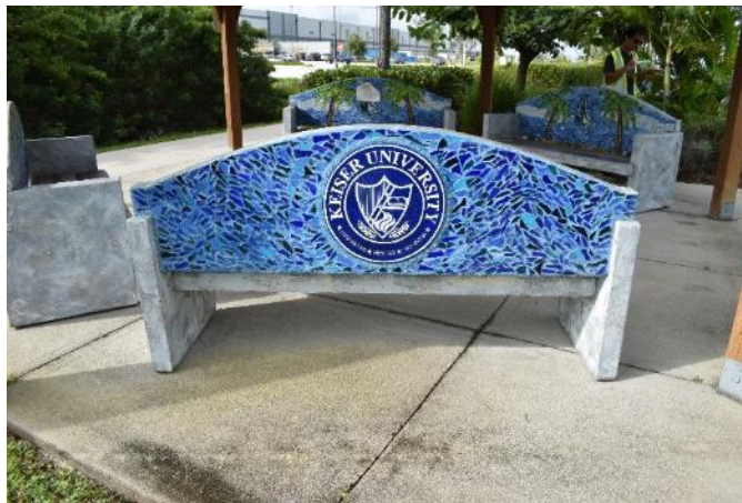
Figure 39. Back detail of the bench (Photo by EverGreene, October 2022).
