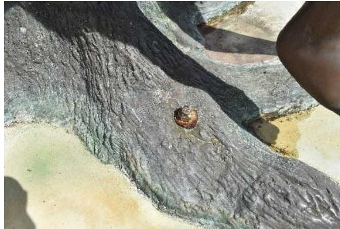
Figure 6. Ferrous bolt supporting the base of the sculpture into the concrete base. The bolt exhibits corrosion and there is apparent staining from the metal sculpture on the surface of the base (Photo by EverGreene, October 2022).
