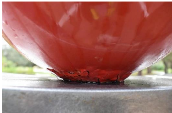
Figure 20. Bottom of the ball with paint peeling from water seepage and corrosion (Photo by EverGreene, October 2022).
