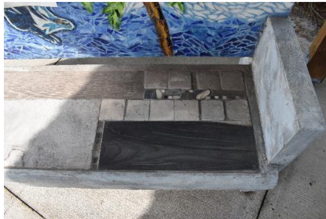
Figure 47. Seat detail of the bench (Photo by EverGreene, October 2022).
