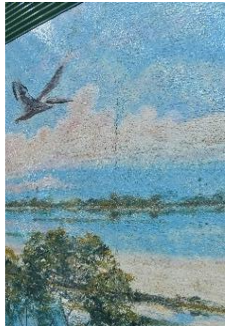
Figure 18. Vertical crack toward the left side of the mural (Photo by EverGreene, October 2022).
