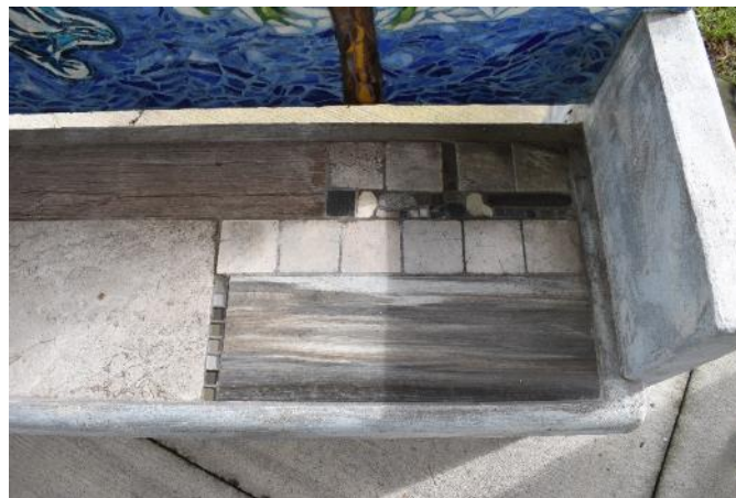
Figure 40. Seat detail of the bench (Photo by EverGreene, October 2022).
