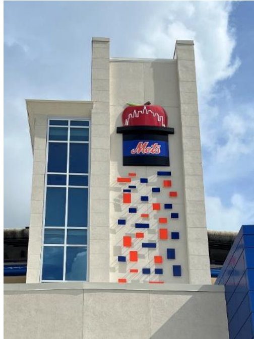
Figure 118. Overall photo (Photo by EverGreene, October 2022).
