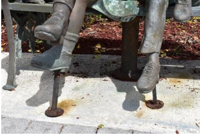
Figure 10. Ferrous support hardware corrosion with residue seeping into the surrounding stone (Photo by EverGreene, October 2022).
