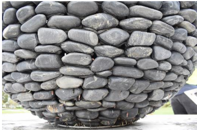
Figure 54. Organic material collected in the gaps between the stones of the sphere (Photo by EverGreene, October 2022).
