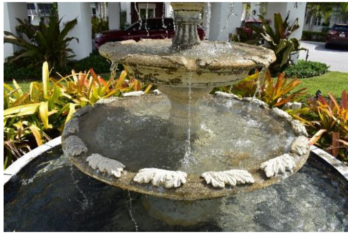
Figure 76. Deteriorated coating on the second and third levels of the fountain. The leaves toward the front of the image appear to have been replaced (Photo by EverGreene, October 2022).
