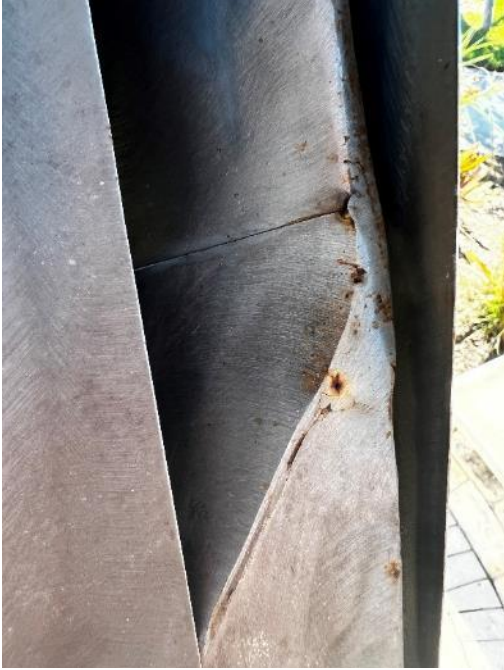
Figure 85. Metal corrosion and broken welds on the surface of the sculpture (Photo by EverGreene, October 2022).
