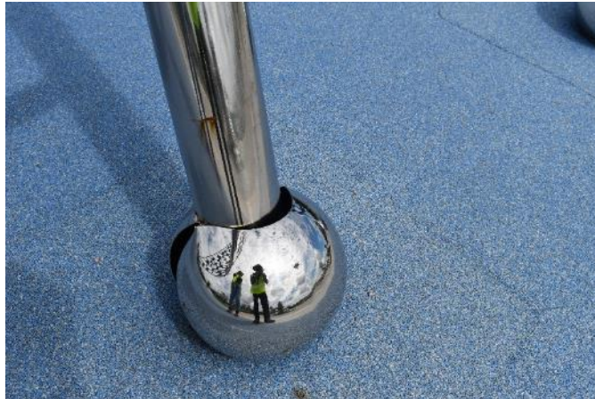
Figure 123. Cracked open ball at the base of one of the sails. There is visible corrosion on the pole extending from it (Photo by EverGreene, October 2022).
