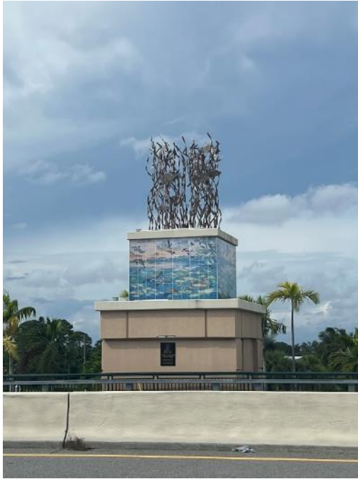
Figure 96. Overall photo (Photo by EverGreene, October 2022).
