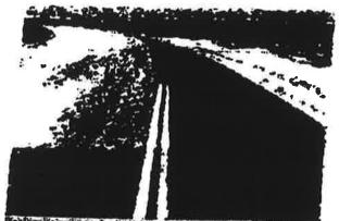
Roblingio was used as a construction seal. For comparison, the lower left area was not treated.
