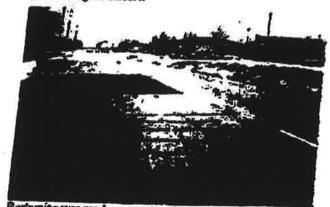
Regismite was used as a construction seal on the dry areas of the pavement. Penetration values of sephall extracted from cores (New Mexico Highway Department).
