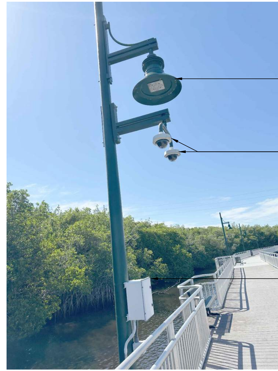
2 EXISTING LIGHT POLE ASSEMBLY w/ SECURITY CAMERAS PICTURE DETAIL
