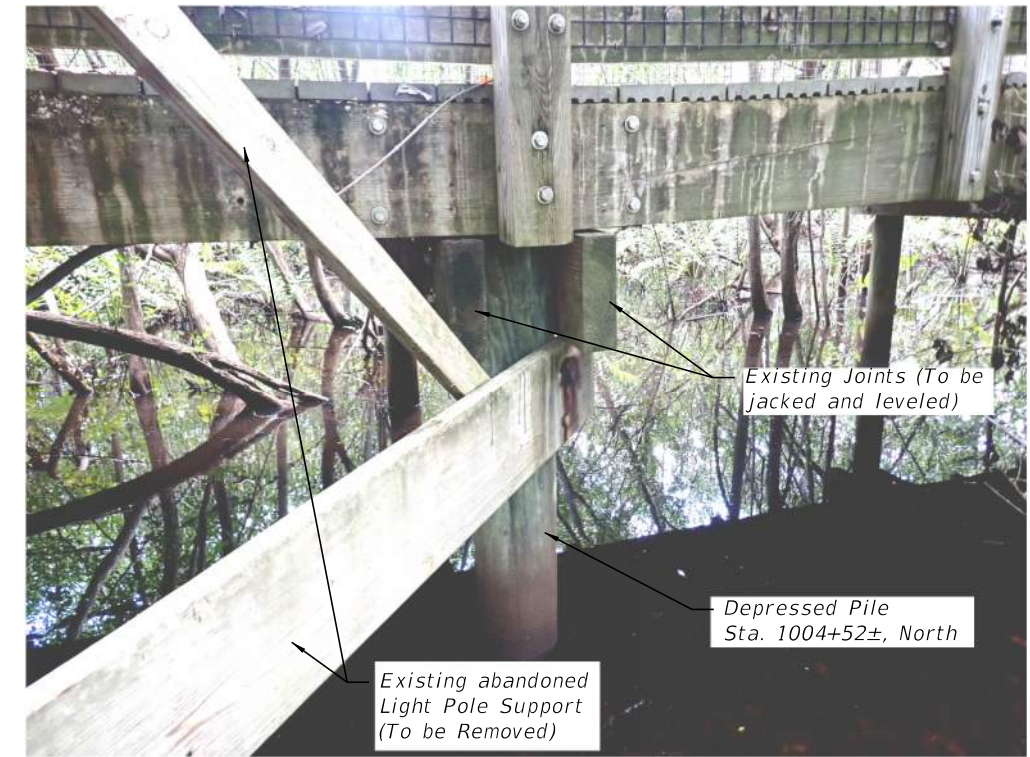
PILE 1004+52± PICTURE (LOOKING SOUTH)
