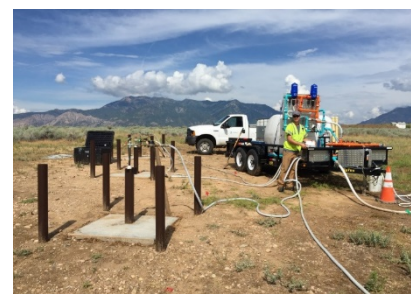
Injecting carbon substrate for bioremediation at Hill Air Force Base, Utah.
