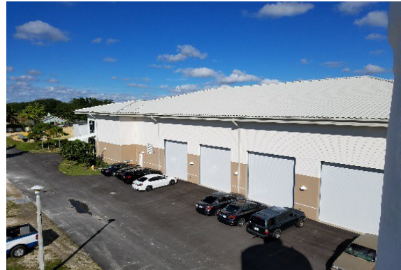
The 11,000 sf membrane building includes process areas as well as offices, control room, laboratory, storage rooms, and operator facilities
