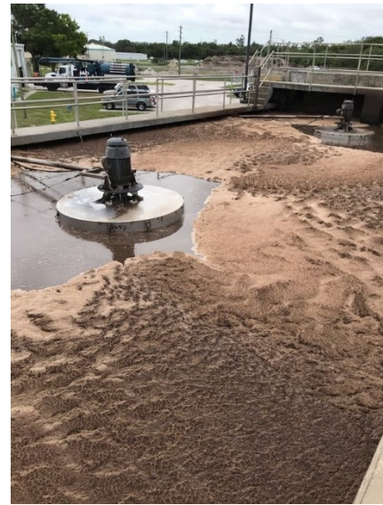
Aerobic Digester at Palm Bay Utilities North Regional WWTP. ISS is performing a Condition Assessment Inspection at all the wastewater facilities as part of the Wastewater Master Plan. ISS will be making recommendations on facilities upgrade needs to be considered for future Capital Improvement Projects.
