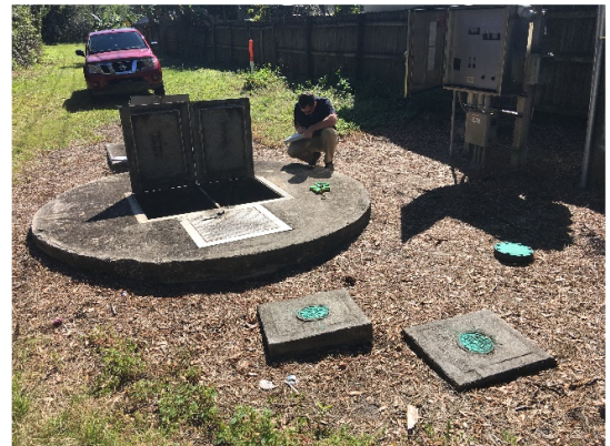
Garrett's Run 10-inch Force Main Replacement
