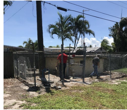
ISS Field Inspection of Existing Palm Bay Lift Station No. 1
