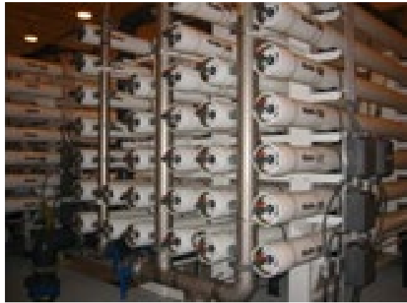
Improvements included New Nanofiltration membrane modules
