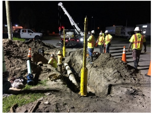
Making the final connections on the Greensboro Force Main project.
