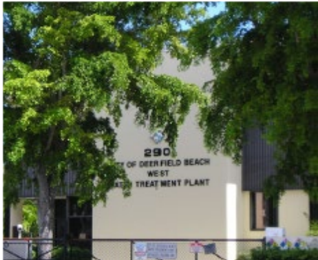
Our team has developed a comprehensive understanding of the City's WTP facilities.
