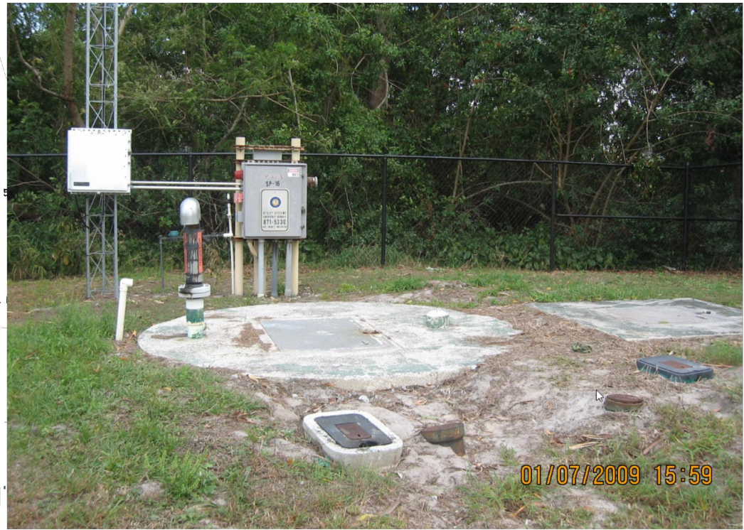
EXISTING CONTROL PANEL, WET WELL SLAB AND VALVE VAULT
