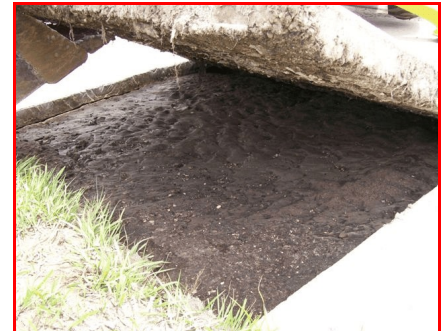
Evidence of soil erosion beneath Adjacent Sidewalk
