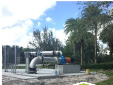
Well Construction, Rehabilitation and Abandonment
