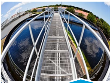
Water, Wastewater and Reclaimed Water Treatment Facilities
