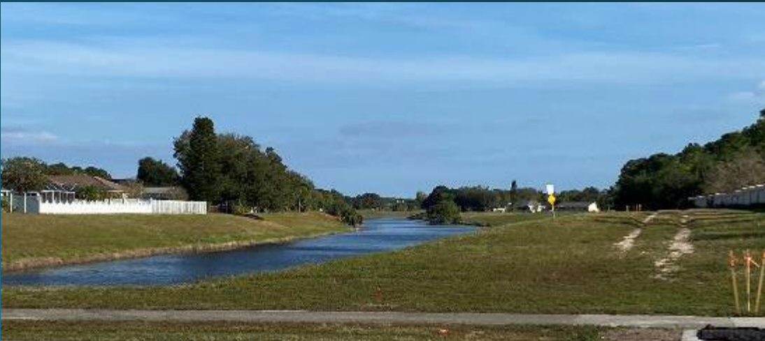
Canals & Drainage Facilities
