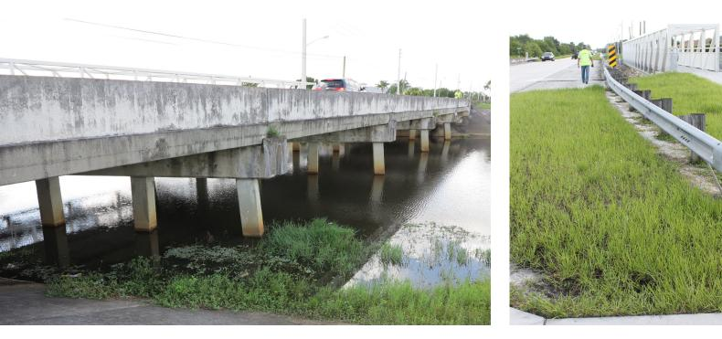
Under an existing continuing contract to provide bridge structural engineering services for the City of Port St. Lucie, GRAEF provided structural engineering services for the rehabilitation of the Darwin Boulevard Bridge over the Canal E-84 (Bridge No. 945262) and analyzed two mast arms located on the NW and SE corners of St. Lucie West Boulevard and California Boulevard.
