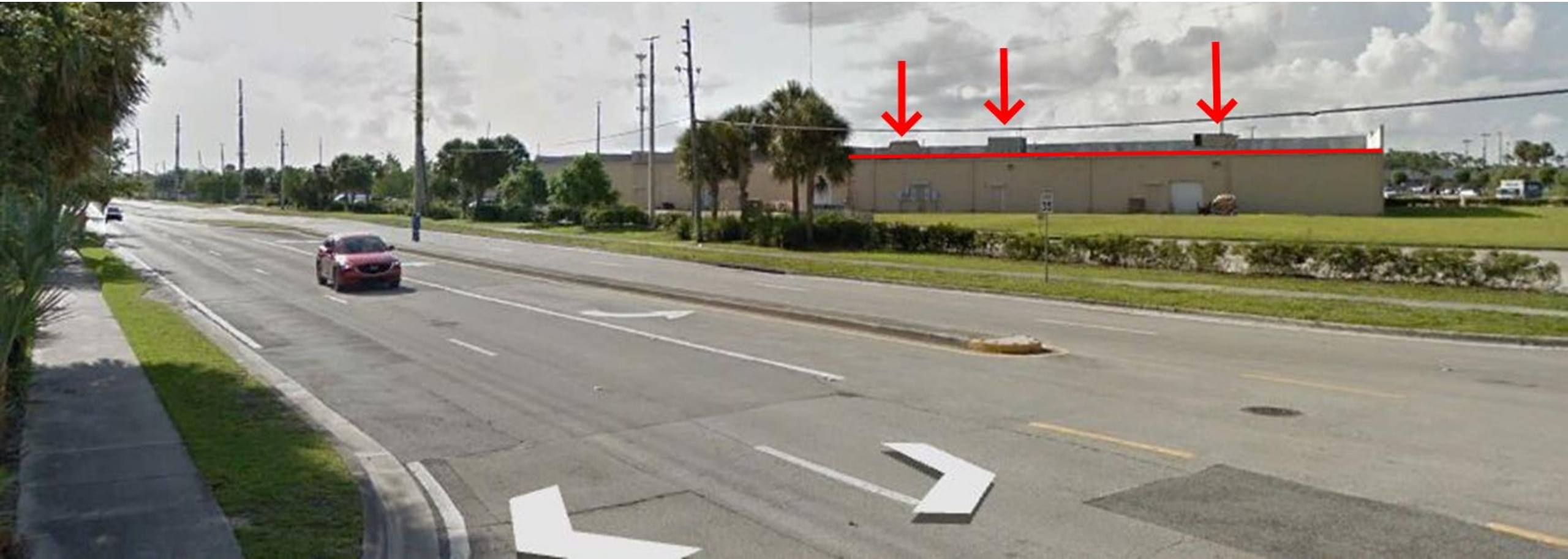
Marketplace Shopping Center on Jennings and US-1. No parapet wall hiding A/C units located on the roof. This distance to building from this location is approximately 300 feet.
