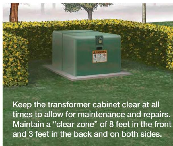
Keep the transformer cabinet clear at all times to allow for maintenance and repairs. Maintain a "clear zone" of 8 feet in the front and 3 feet in the back and on both sides.
