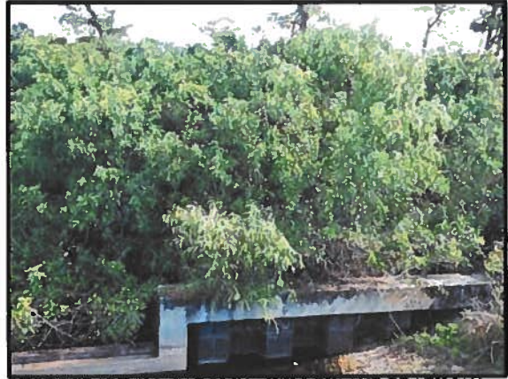
PHOTOGRAPH #26: CAROLINA WILLOW AND BRAZILIAN PEPPER BEHIND A-24 WEIR, FACING NORTHEAST.
