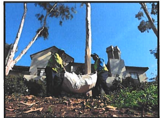
Use two-man method to haul debris down a slope
