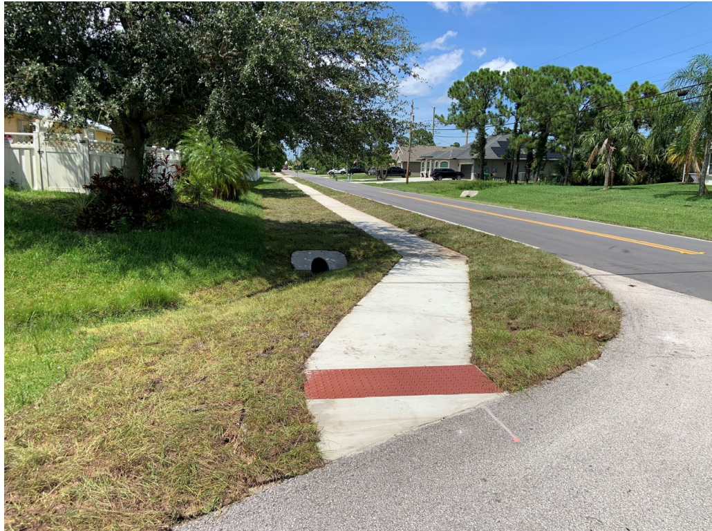
Brescia Sidewalk: Complete From SW Gatlin Blvd. to SW Savage Blvd.
