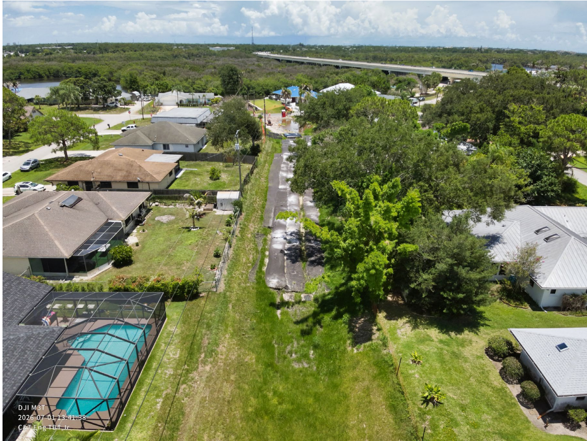
Floresta Drive Phase 3 – D-11 Canal Activities
