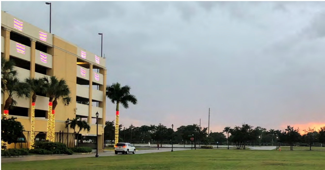
Figure 28 Image of the existing 900-space parking garage funded through the special assessment district.
