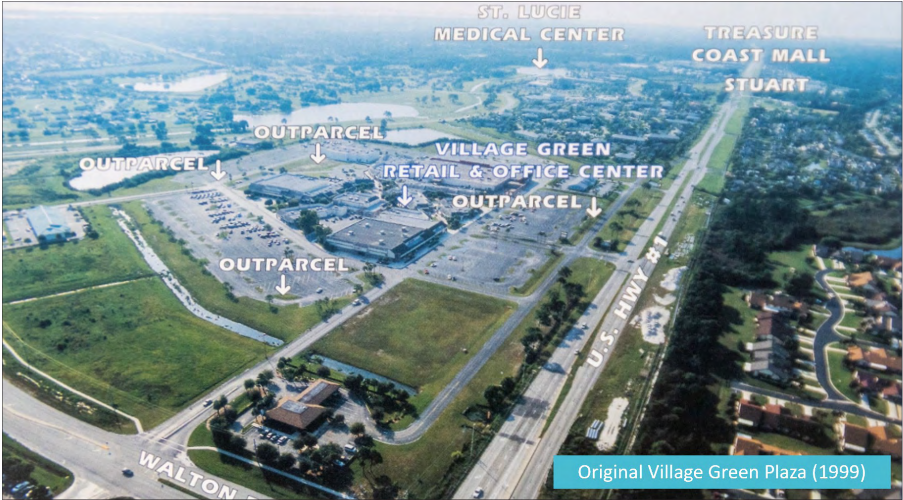
Figure 20 Aerial photo of original Village Green Plaza property c1999
