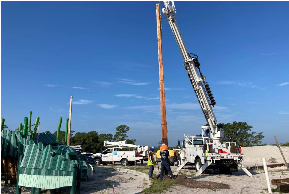
Featured Photo: Construction at Pioneer Park at The Port
