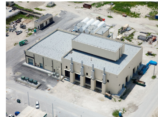
Miami-Dade Water and Sewer Department, South District High-Level Disinfection Program $618 million
