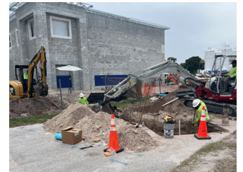
City of Stuart Water Treatment Plant Reverse Osmosis Treatment Facility $16.7 million
