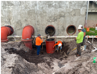
1021-562 City of Port St. Lucie Westport WWTF Expansion Phase $2.2 million
