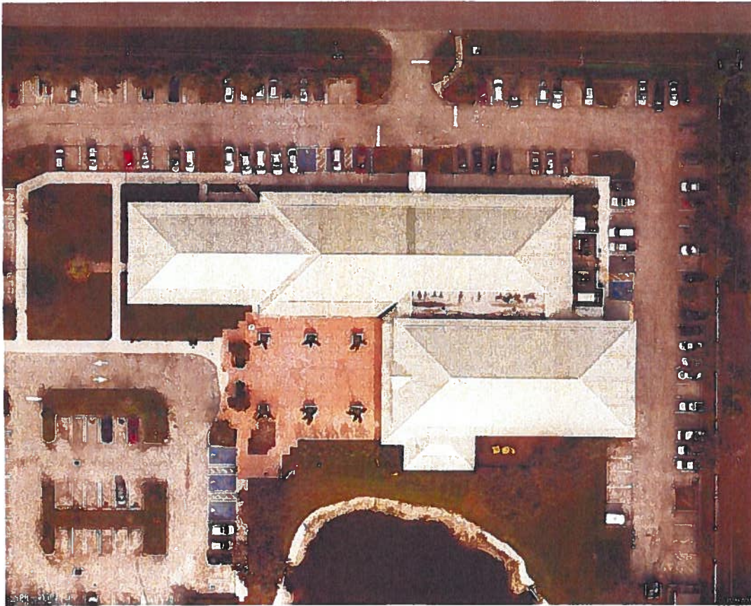
Roof Section Photo
