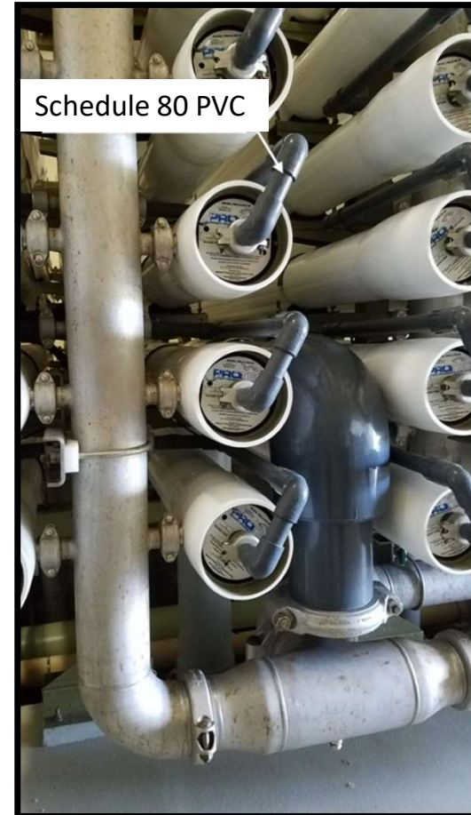
1.25" Permeate Piping and 1/2" Sample Valve. Skids 1-3 (Left). Skids 4-10 (Right)
