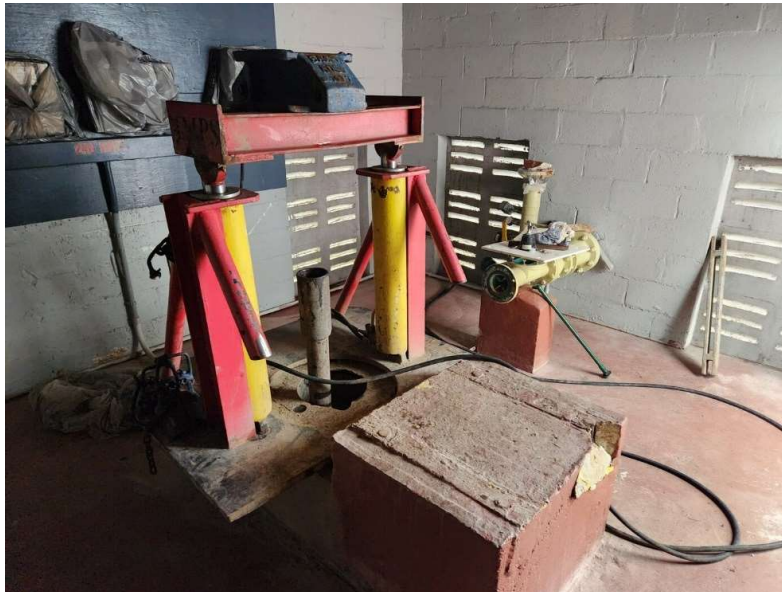
Photograph 1 – Well #12 with drill pipe extended above rigging plate
