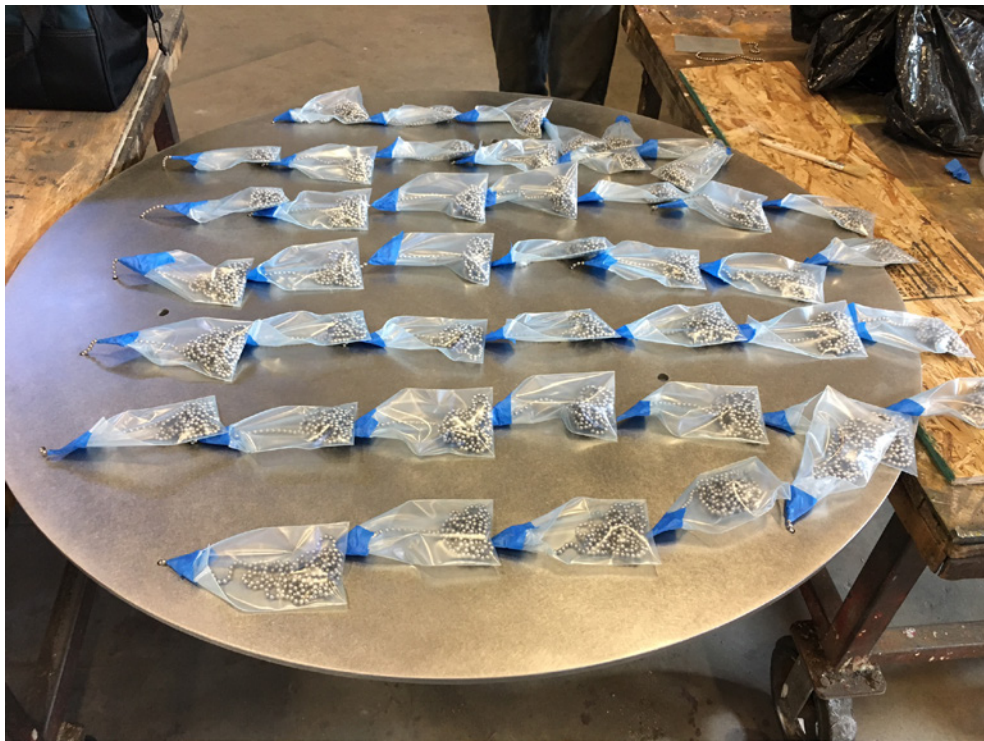
Base plate pre-drilled with beadchain installed prior to sculpture installation. Base plate installed by contractor on site to pre-determined ceiling mounting hardware.
