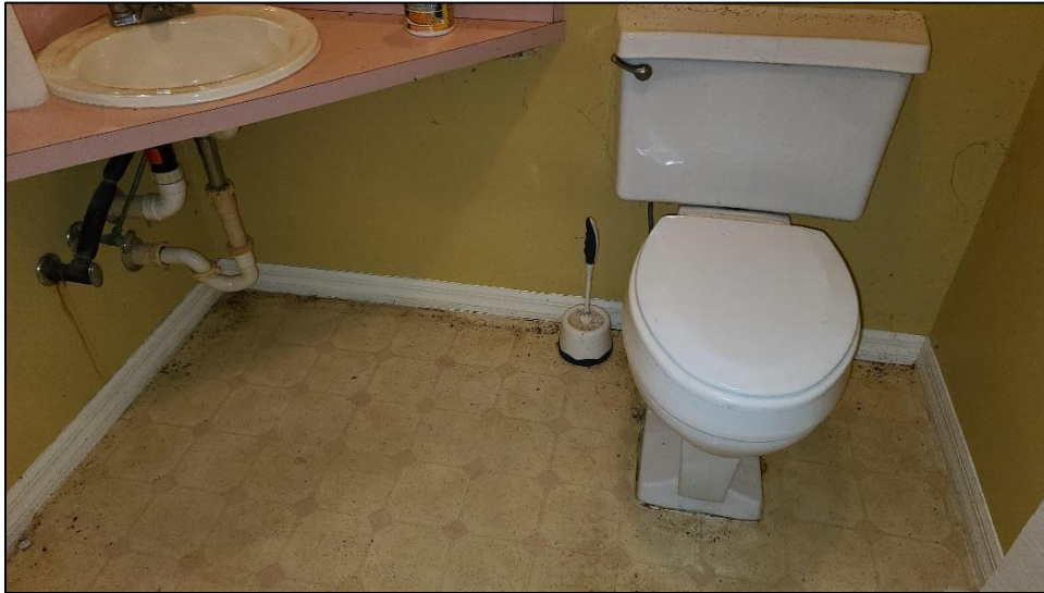
VIEW OF TYPICAL BATHROOM
