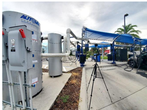
Figure B2. Photographs of the vacuum producer and vacuum stations at Joe's Express Carwash in Clermont, Florida.
